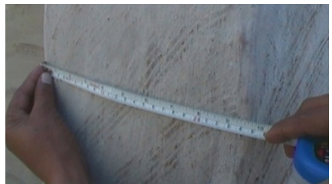
Figure 4: Mud wall 450mm thick. (Source: Clicked by author).
