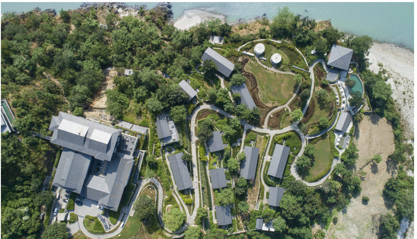
Aerial view of Taj Resort and spa, Himalayas (Source : Edifice consultants)
