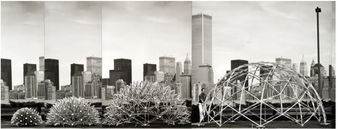
Image 6: Deployable dome by Hoberman
