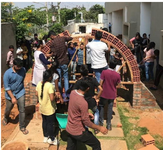
Fig 4: Process of construction of Masonry vault (Source : Author)
