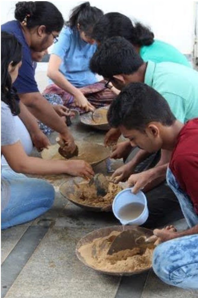
Fig 6– Students preparing batches of natural plaster (Source : Author)
