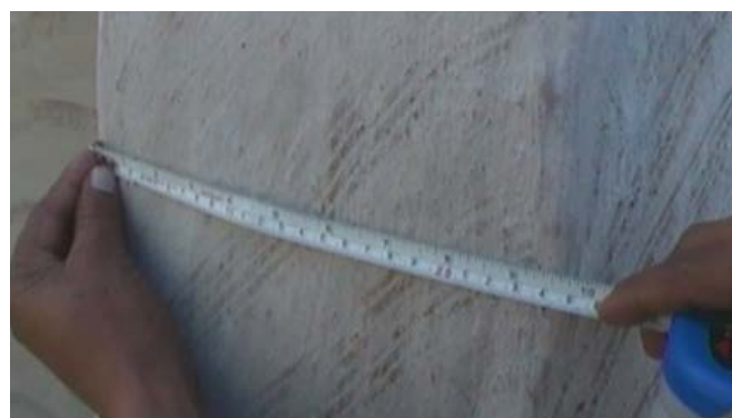
Figure 4: Mud wall 450mm thick. (Source: Clicked by author).
