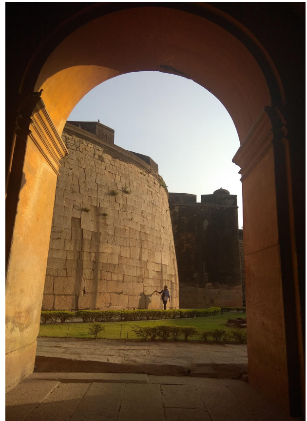
Figure 2. Inside Bangalore Fort
