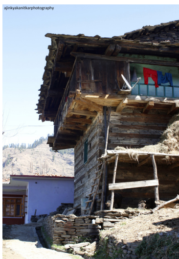
Figure 3: Typical Kathkuni house- animal shed at base, living areas at the upper levels with cantilevered rooms
