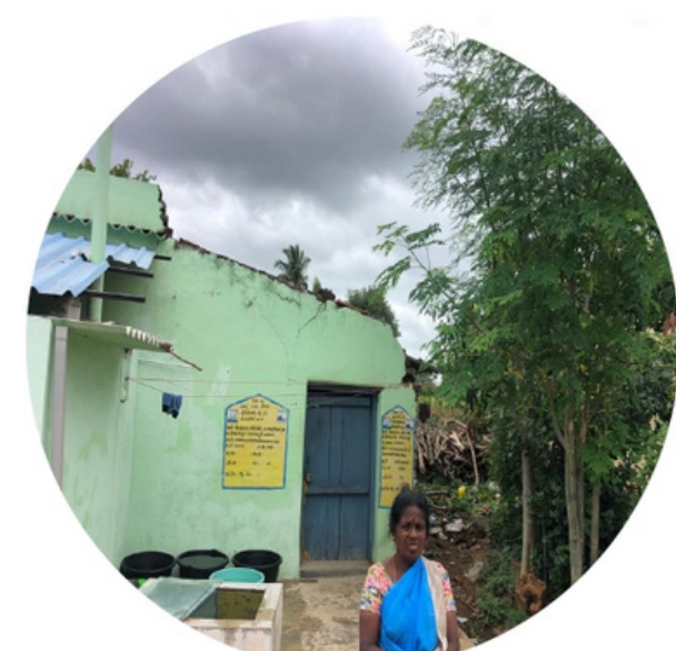
HALF DEMOLISHED HOUSE
