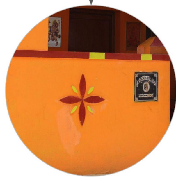
LOCAL MOTIFS, PATTERNS, OR DESIGNS ON WALLS CAN REFLECT THE COMMUNITY'S UNIQUE IDENTITY AND CREATIVE HERITAGE.
