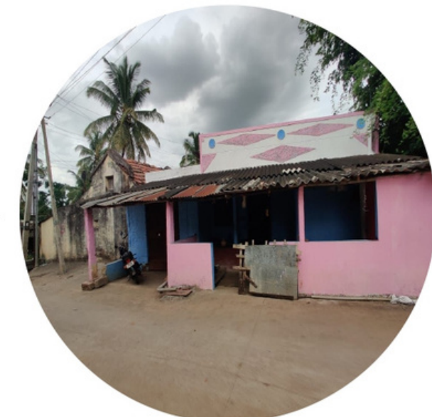
A SMALL HOUSE WITH A FRONT PORCH HAVING A MANGALORE TILED LEAN TO ROOF.
