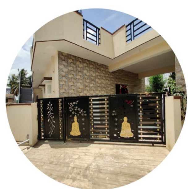
ONE OF THE FEW RECENTLY BUILT HOUSE IN THE LOCALITY
