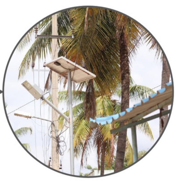
OUT OF ALL THE STREETLIGHTS IN THE VILLAGE, THIS IS THE ONLY ONE THAT WAS SOLAR POWERED. IT SHOWS AWARENESS AND AN EFFORT TOWARDS USING RENEWABLE ENERGY.
