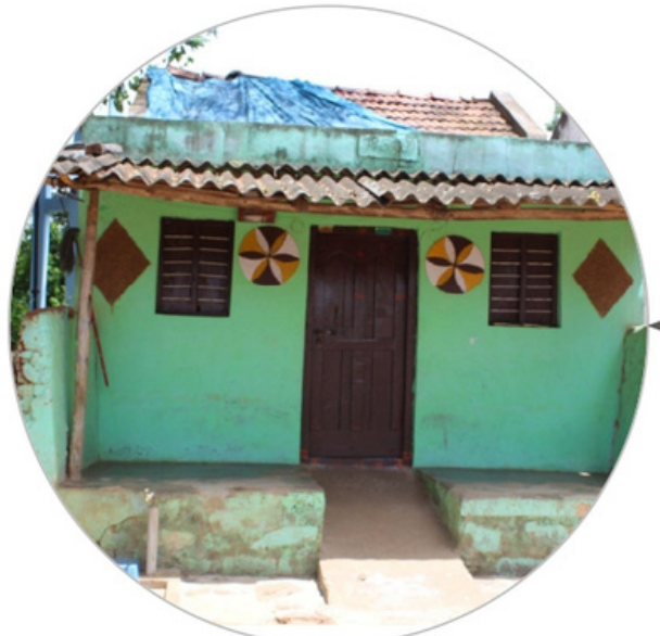
HOUSE WITH DECORATIVE EXTERIOR
