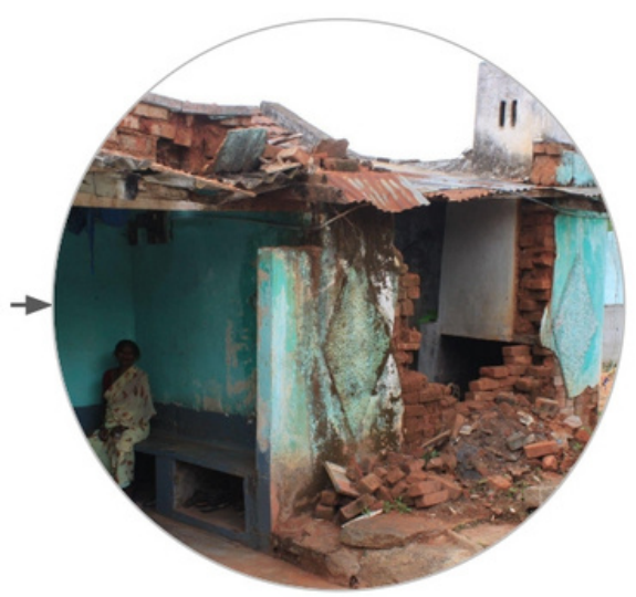
THE NUMEROUS RANSACKED HOUSES IN THE VICINITY OF THE SITE DEPICTS THE VULNERABILITY OF THE STRUCTURES TO HEAVY MONSOON WINDS AND RAINFALL
