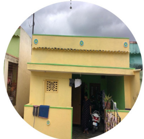
HOUSES HAD LINTELS AT VARIOUS HEIGHTS JALIS FOR VENTILATION AND LIGHTING CAN BE FOUND IN MANY HOUSE
