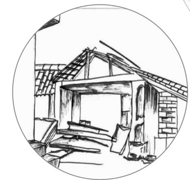
A VERY OLD DEMOLISHED HOUSE WHICH HAS U-SHAPED TILE ON THE ROOF A COMMON PLACE USED BY THE PEOPLE OF THE LANE TO DRY CLOTHES
