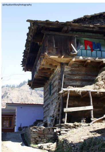
Figure 3: Typical Kathkuni house- animal shed at base, living areas at the upper levels with cantilevered rooms
