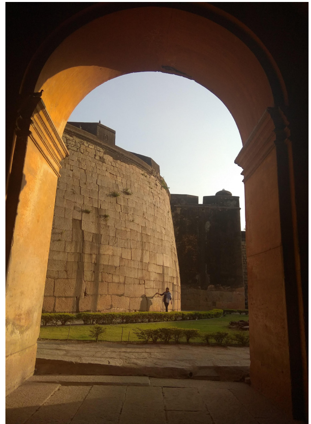
Figure 2. Inside Bangalore Fort
