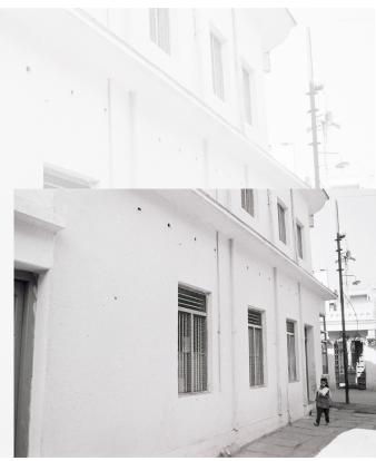
Even in 1987, the traditional morphology was in flux, and this 19<sup>th</sup> century house was a rare holdout. Timber columns, beams and purlins supported a brick 'Madras terrace' roof. The low plinth level indicates how much the road surface was already raised, a sure sign of development. Land values demand three-four floor walk-ups, so concreteframed structures are the default. They now house businesses now that deal in a gamut of goods, from watch parts to toys to tailoring accessories.
