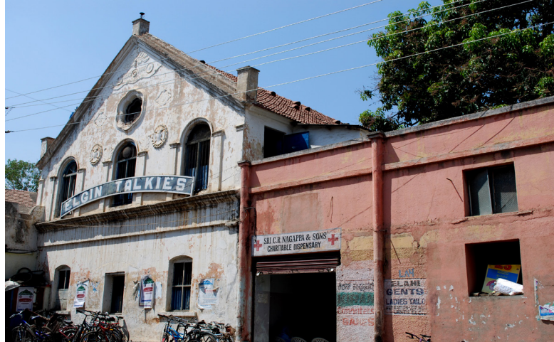
Elgin Talkies, Hazrath Kambal Posh Road, Shivajinagar (Source: Aliyeh Rizvi)
